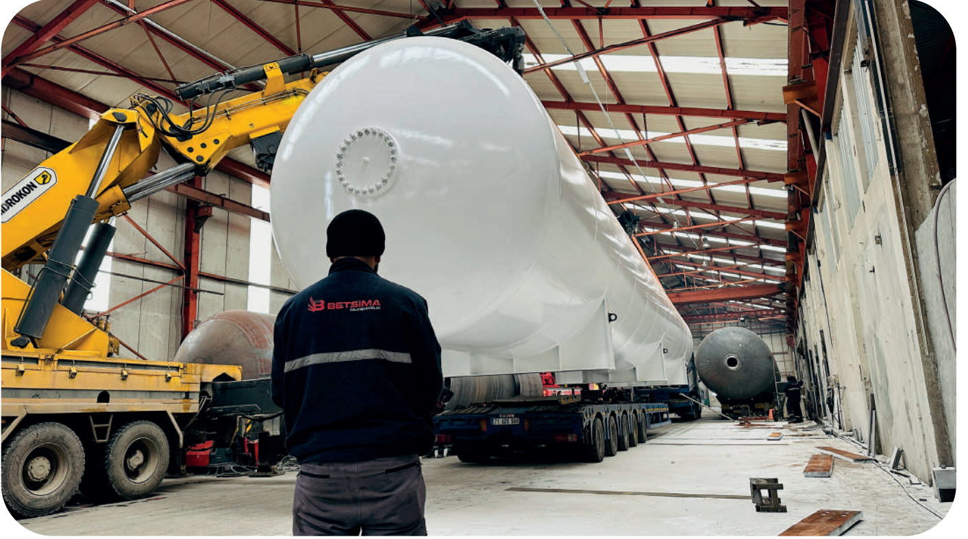
250m 3 Stok Tankı / Storage Tank
